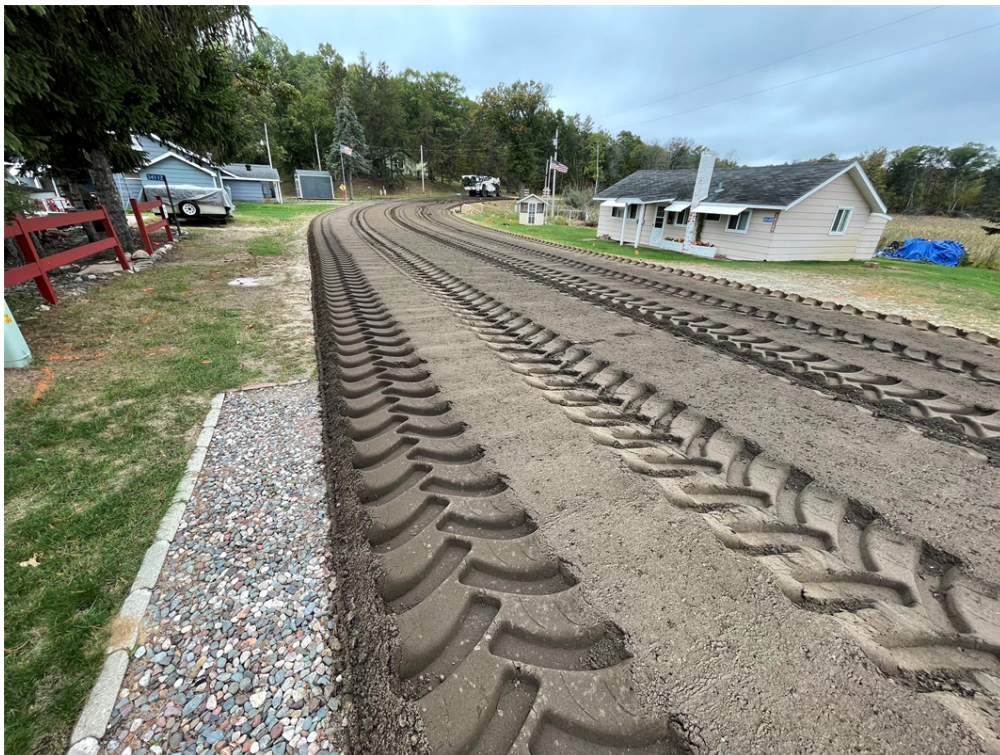
Photo #5: Milling Aztec Road - Sep 29, 2023, 2:45 PM
