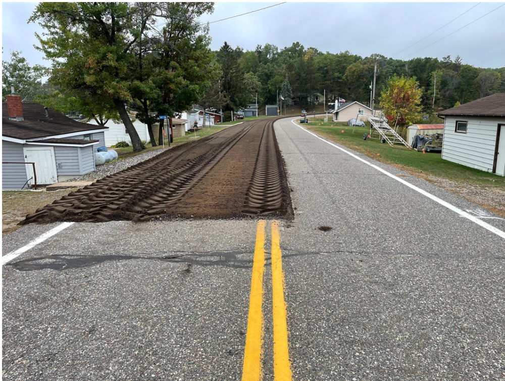
Photo #1: Milling Aztec Road for removal - Sep 29, 2023, 2:33 PM
