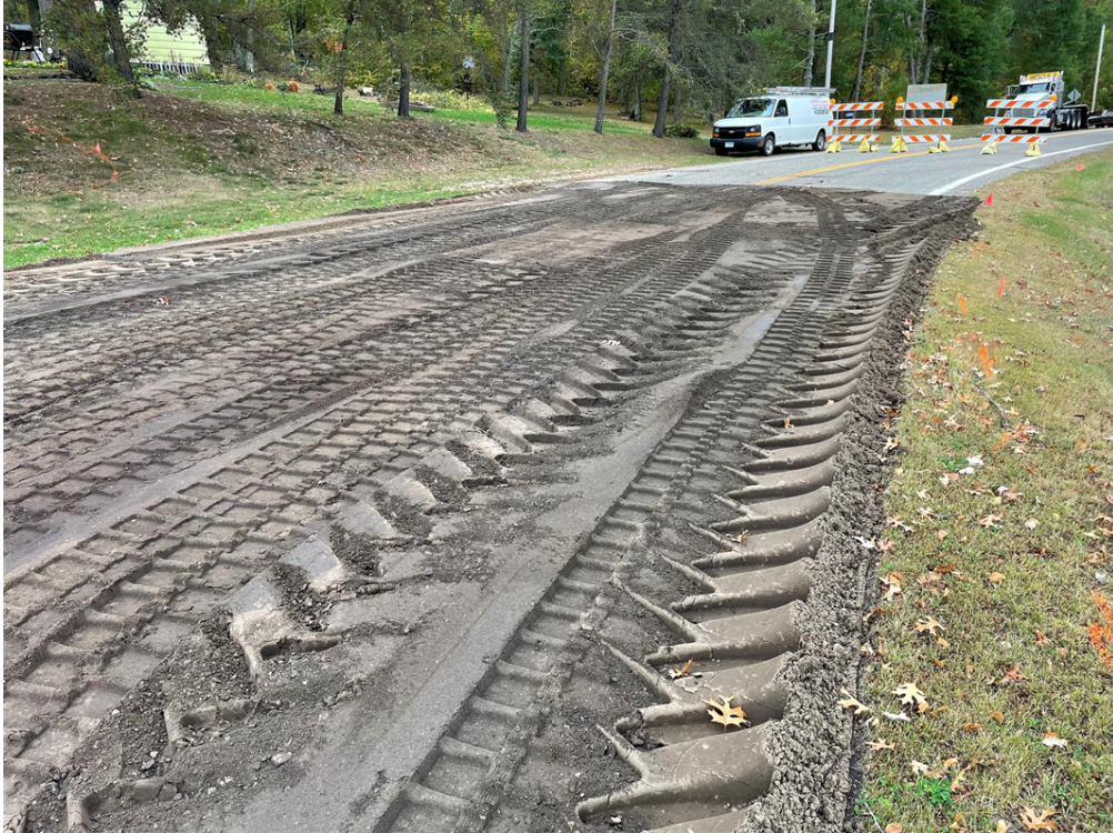
Photo #6: Traffic Control Barricades - Sep 29, 2023, 2:47 PM
