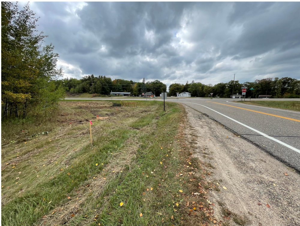
Photo #3: Clearing and grubbing the right-of-way Aztec Road - Sep 29, 2023, 2:35 PM
